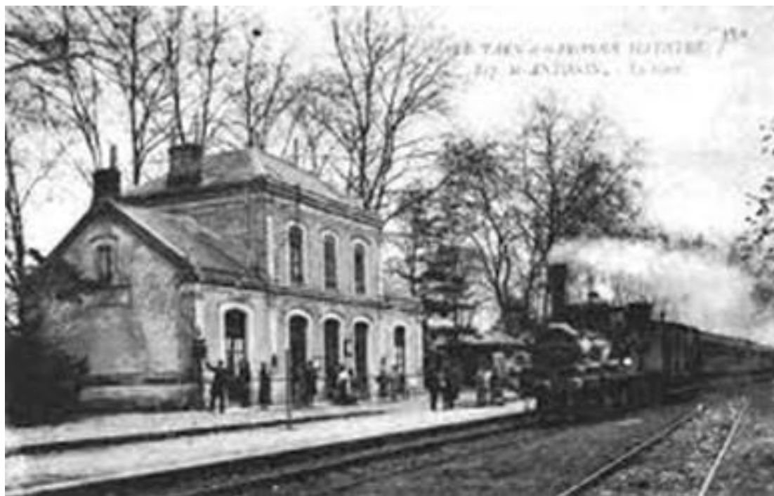
Figure 6. The station at St Antonin-Noble-Val in 1895 4
